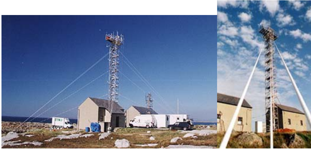
Figure 5 The original 22 m AEROCE tower and the 2 shore laboratories
