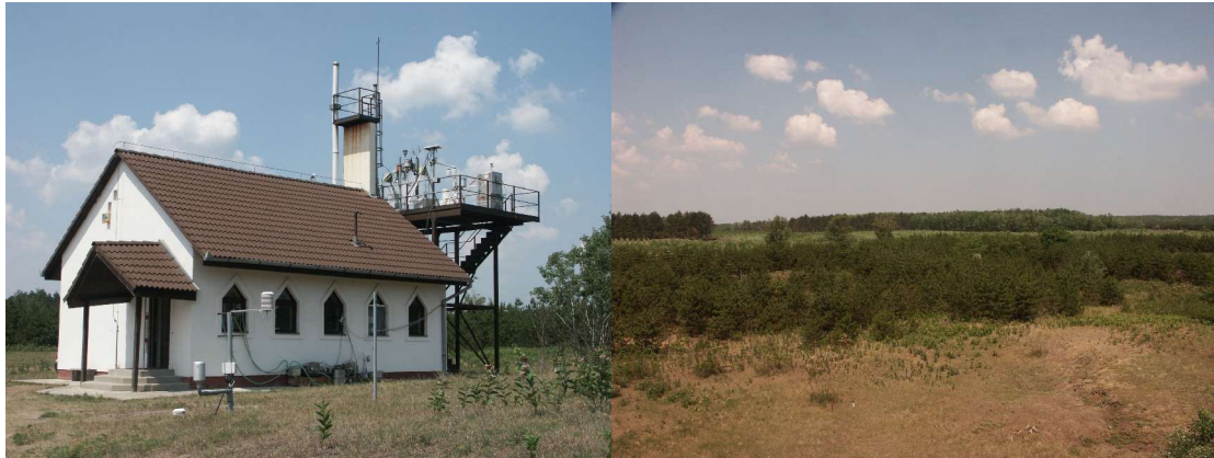
1. The K-puszt station
