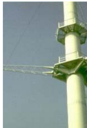
9.4 m booms at 20 m in directions
